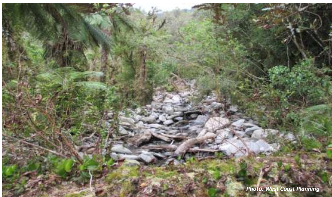
Figure 8: Alpha Creek looking upstream at a confined point where the creek bed exits cliffs ( works to occur from the channel at the base of the cliffs down to the tailrace ).
