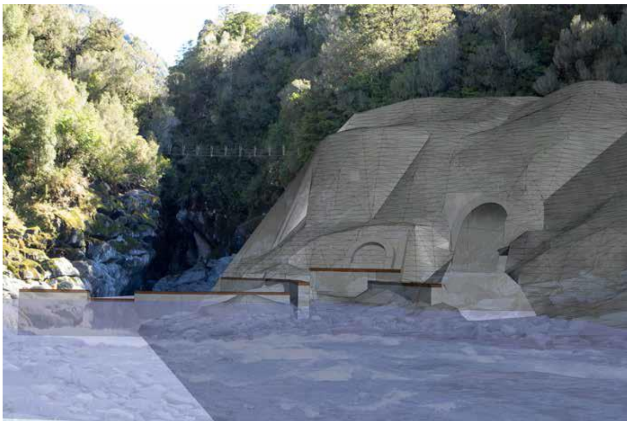
Intake Structures - IN1 April 2016
