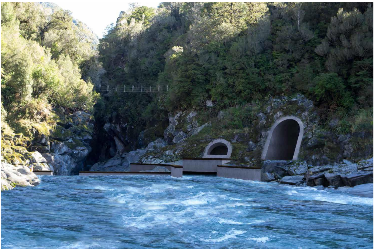
Intake Structures – IN1 April 2016
